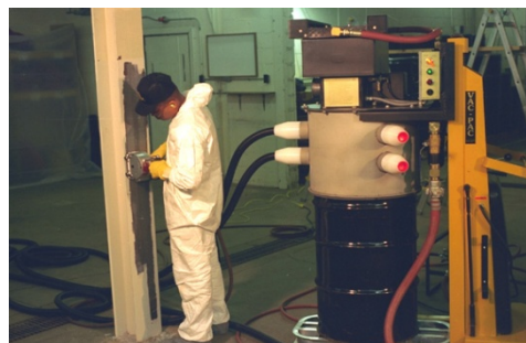
Worker is using the roto-peen (scabbler) attachment; VAC-PAC collection system shown with 55 gal drum.
